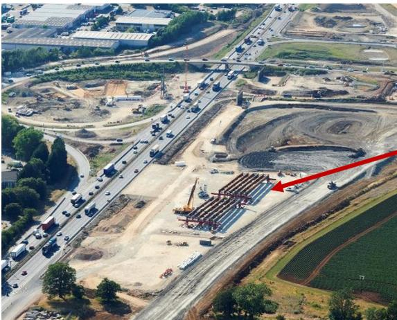
The side sections “abutments” for the new bridges at Bar Hill are progressing well and the steel girders which will span the A14 and form the bridge for the new junction can be seen resting beside the east-bound carriageway, as pictured. We expect to lift these beams into place in September, when there will be a Friday night to Monday morning closure of the A14.
